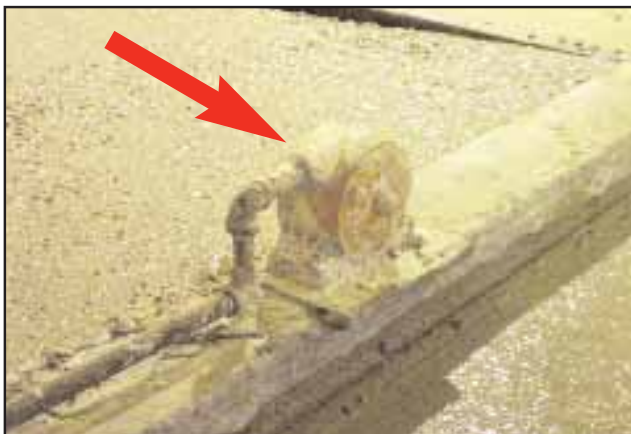
VS-510 SILENT TURBINE VIBRATOR ON CONCRETE SCREED eliminated blemishes from ball vibrator lubricant leaks and reduced noise levels significantly.
